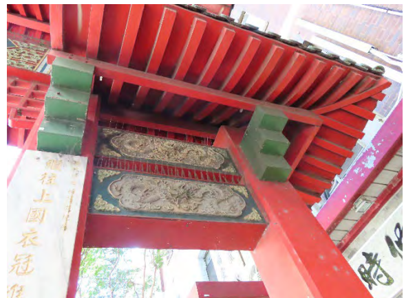
Figure 4.11 Underside of curved timber rafters and plywood soffit on the lower roof.
