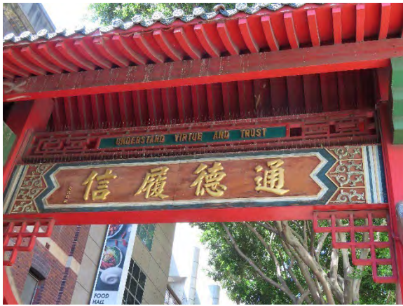
Figure 4.4 Panels A and B on north elevation with inscription in English above and Chinese below: 'Understand virtue and trust'. Decorative lattice brace C beneath panel B.
