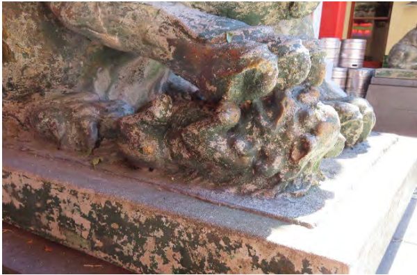
Figure 4.51 Poor condition of the painted concrete lion.
