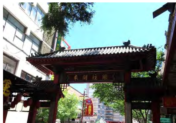
Figure 4.3 South elevation (image taken from the south).
